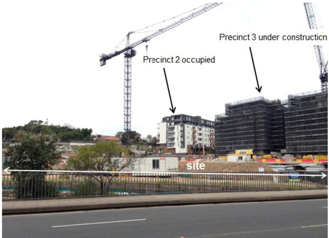
Figure 3: Site viewed from The Crescent looking east
