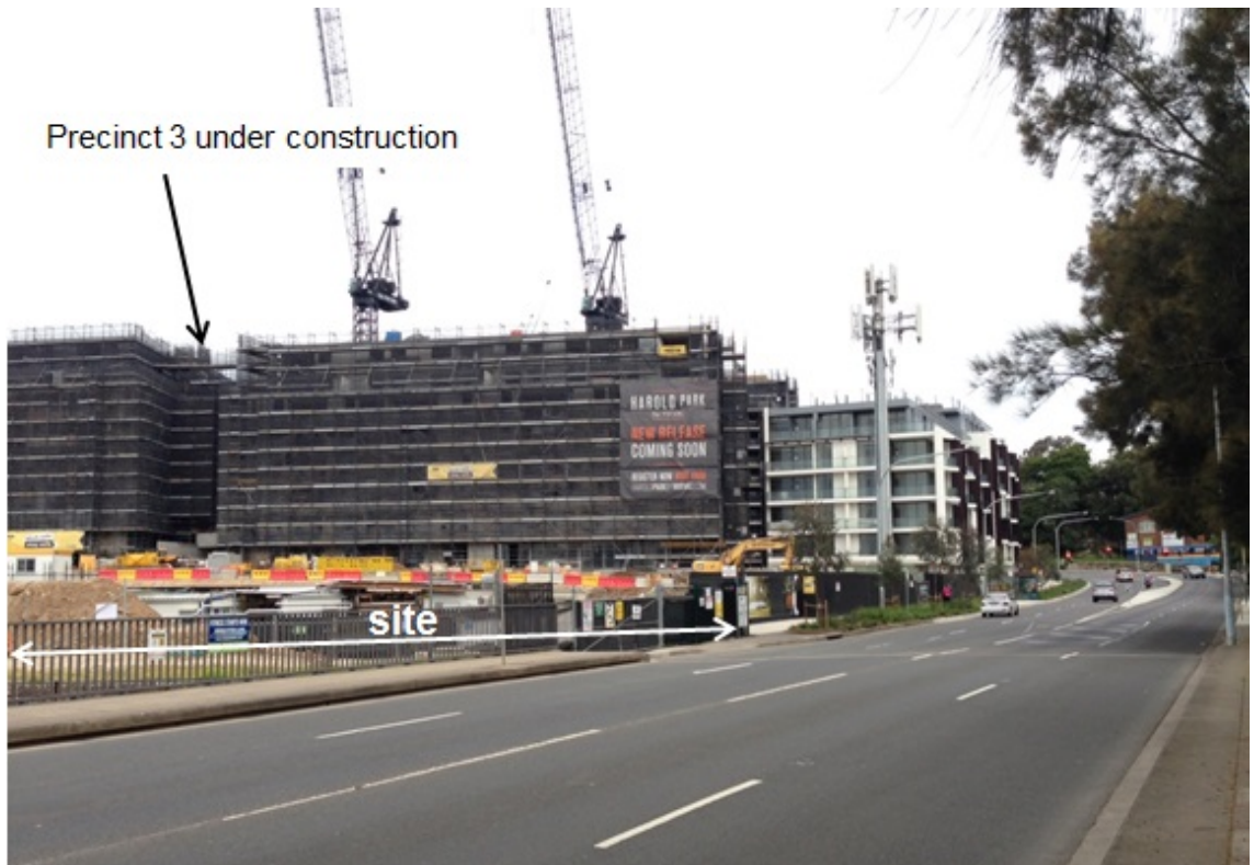
Figure 4: Site viewed from The Crescent looking south east
